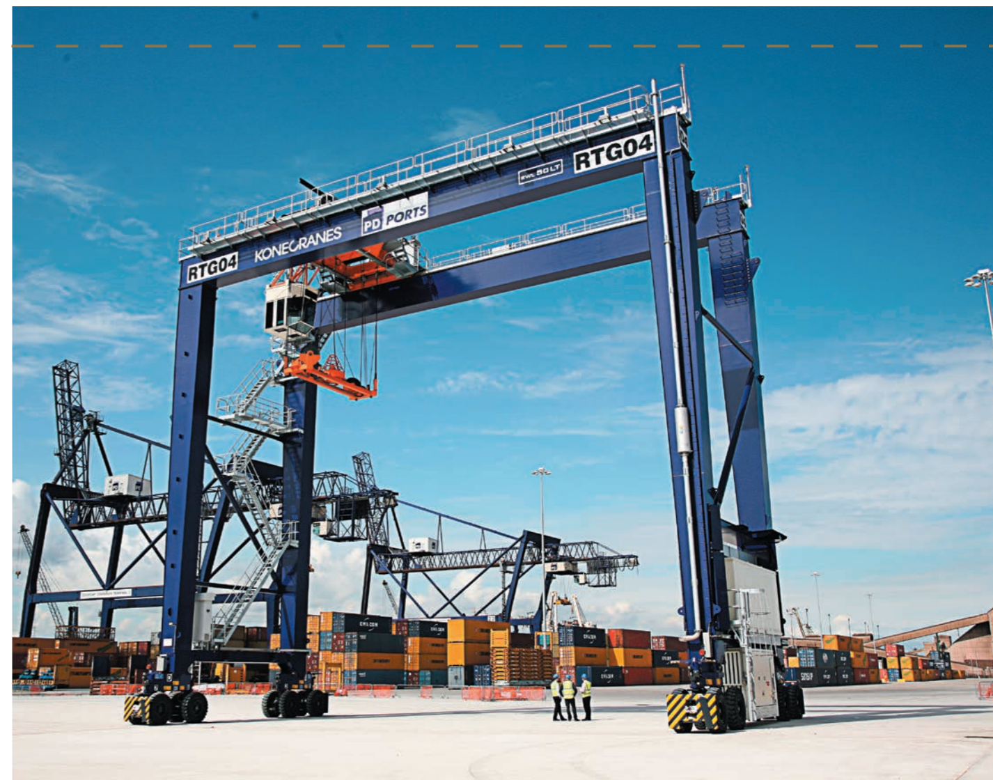
Installation of new RTG cranes at Teesport Container Terminal 2, August 2011
